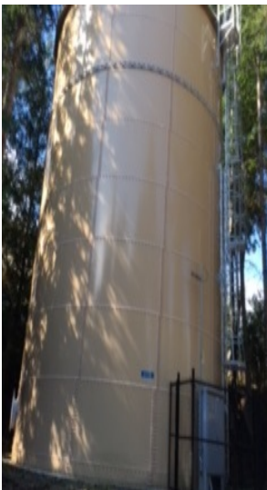
165,000 gallon tank on Frigate Road
