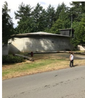
Trincomali's 300,000 gallon storage tank
